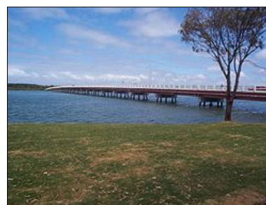
Bribie Island Bridge
